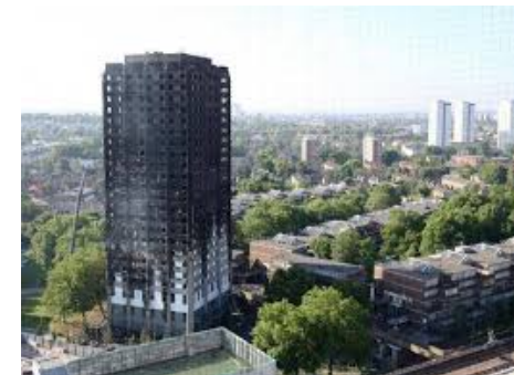
Grenfell Tower, London, 2017
